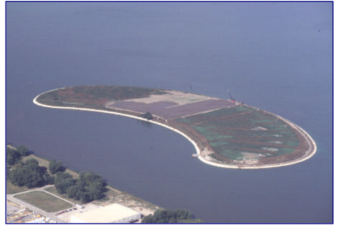
Confined Disposal Facility
